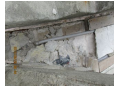
Deteriorating sloped roof stone
