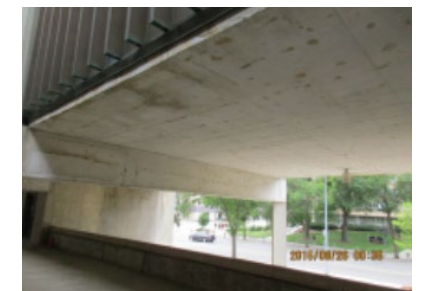
Uninsulated, unheated elevated floor slabs
