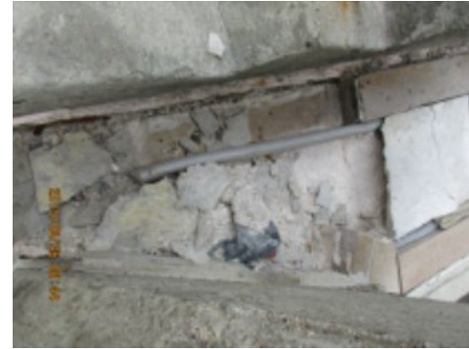
Deteriorating sloped roof stone
