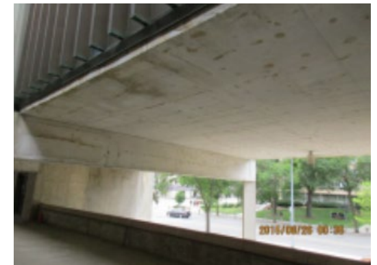
Uninsulated, unheated elevated floor slabs
