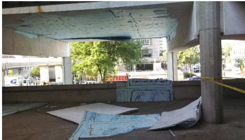
2013 Ceiling Collapse over outdoor deck
