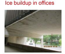
Uninsulated, unheated elevated floor slabs
