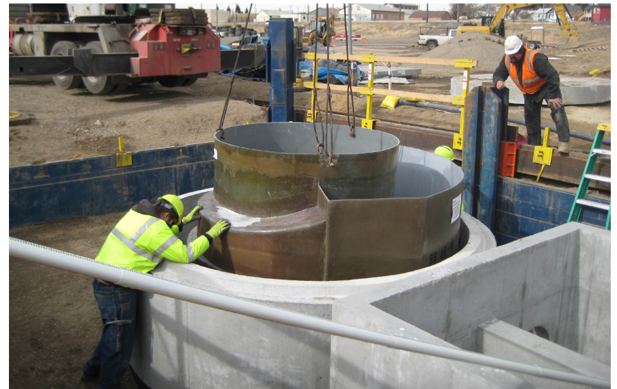
Figure 5-48 Installation of a Hydrodynamic Device, Butte, Montana
