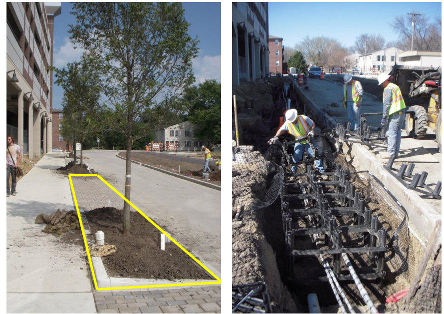
Figure 5-53 Installation of Silva Cell Root Enhancement Zone
