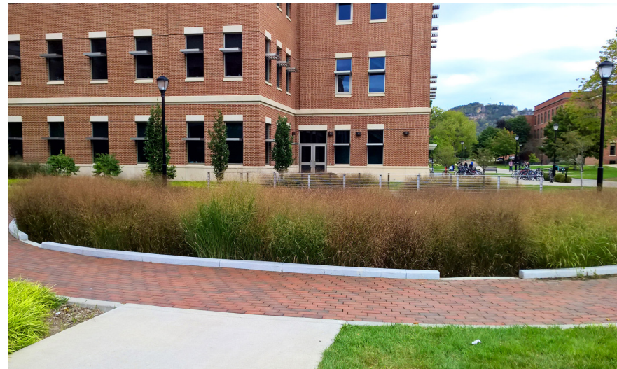
Figure 5-23 Biofiltration Area at Centennial Hall, UW-La Crosse
