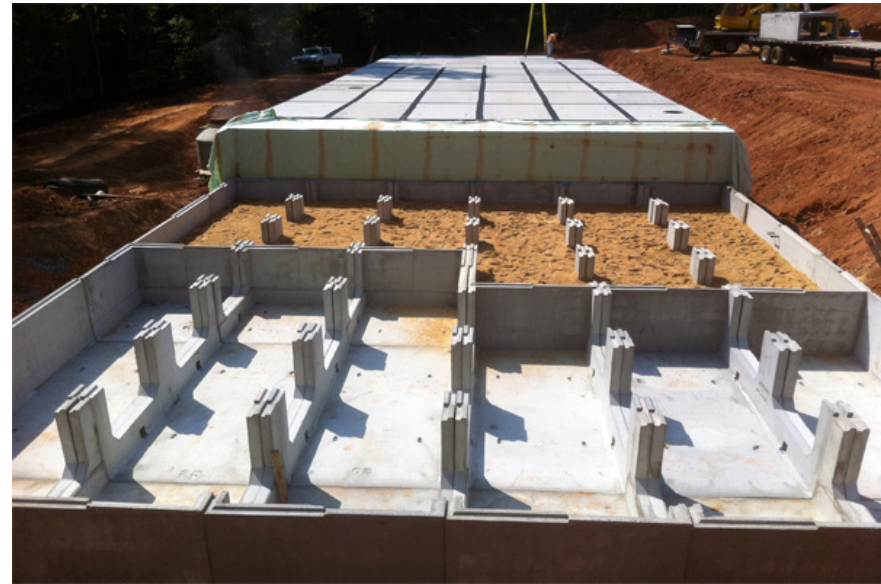
Figure 5-13 Underground Detention Precast Units Being Installed
