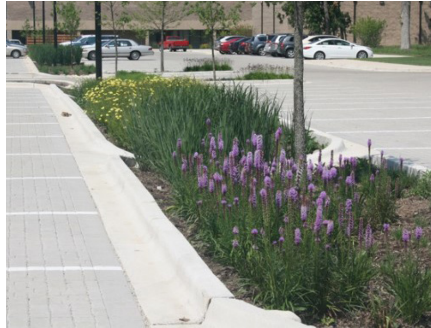
Figure 5-5 Parking Lot Median Bio Filters
