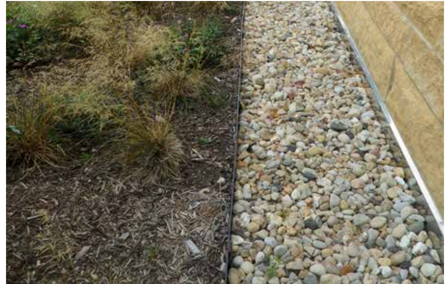
Figure 128 Standard Aggregate Maintenance Strip with Steel Edging
