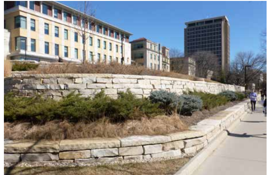
Figure 120 Natural Limestone Retaining Wall
