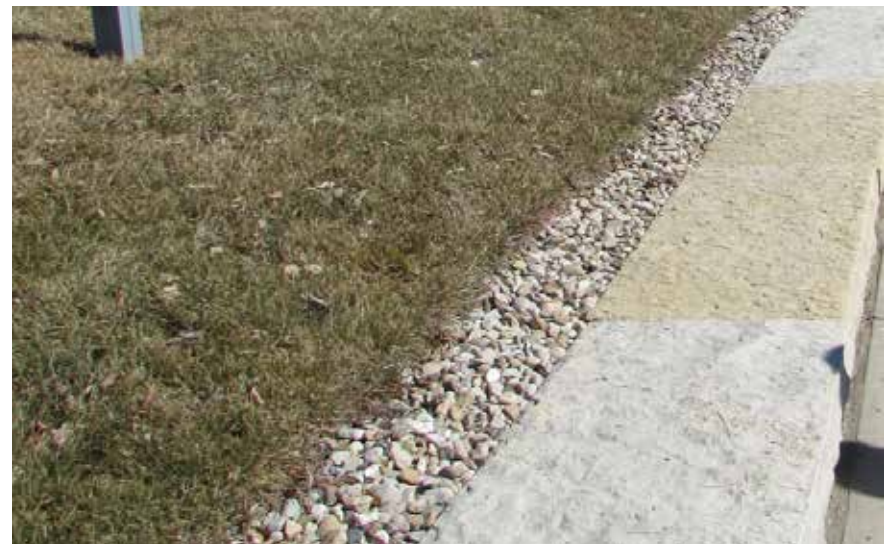
Figure 129 Aggregate Maintenance Strip between a Stone Retaining Wall and Lawn
