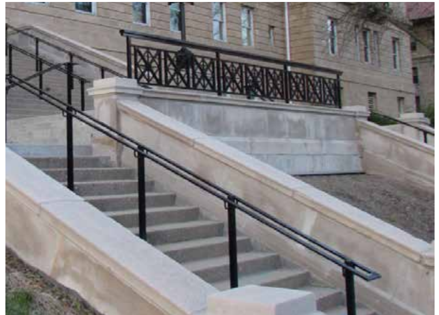
Figure 156 Unified Guardrail and Handrail Design
