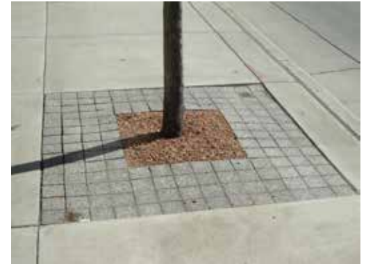
Figure 143 Granite Tree Pavers
