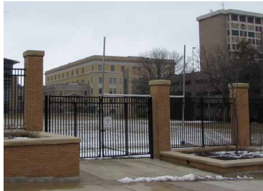
Figure 148 Typical Campus Black Ornamental Fence and Pier Masonry
