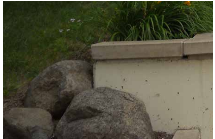
Figure 163 Decorative Boulders at Wall Terminus
