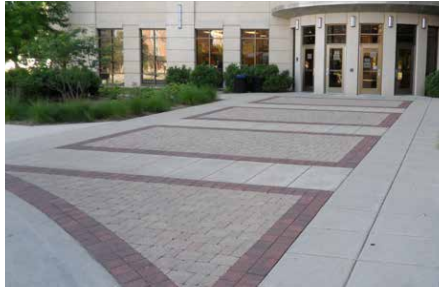
Figure 113 Concrete Unit Pavers are Preferred in High Traffic Areas
