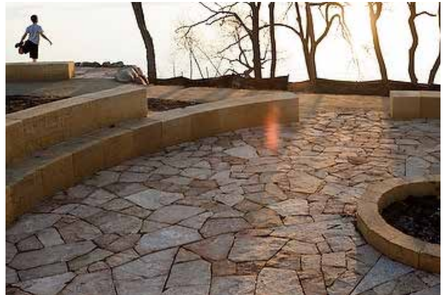
Figure 116 Flagstone Paving at Picnic Point
