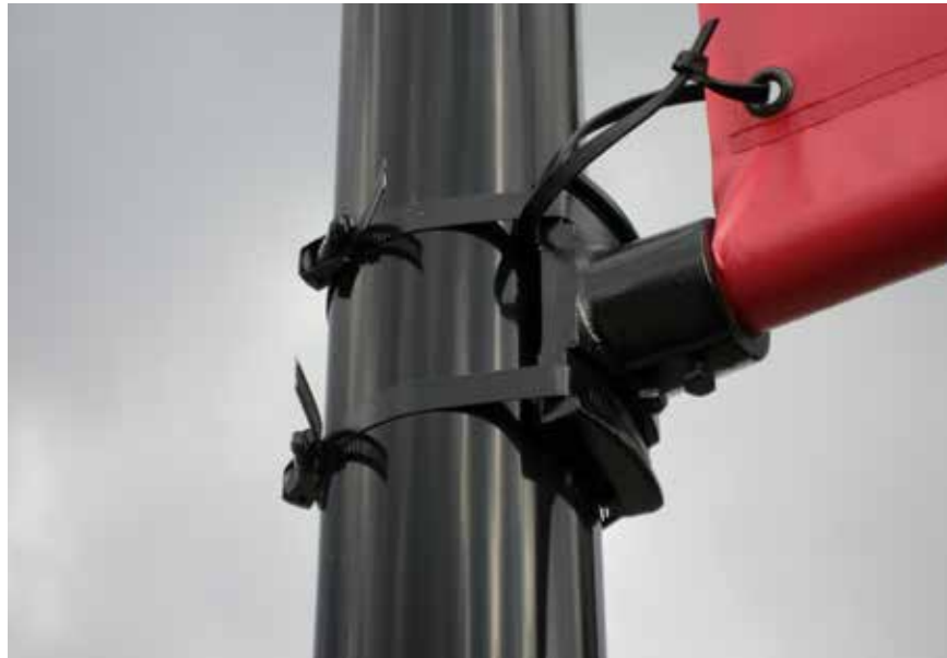
Figure 171 Banner Post Mounting Connection
