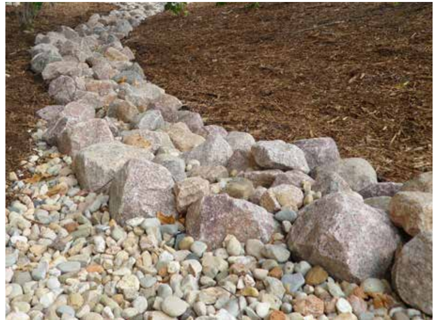
Figure 160 Granite Cobble Rip-Rap
