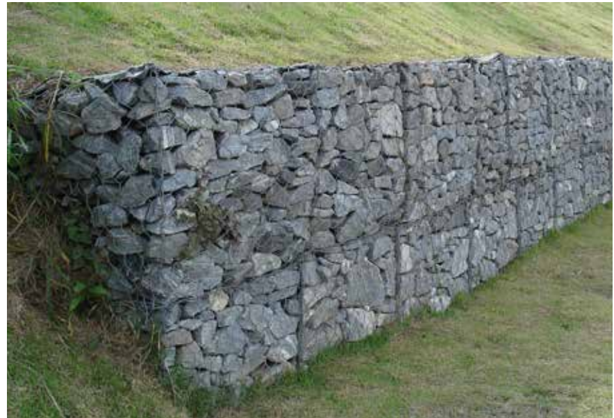
Figure 123 Gabion Stone Wall
