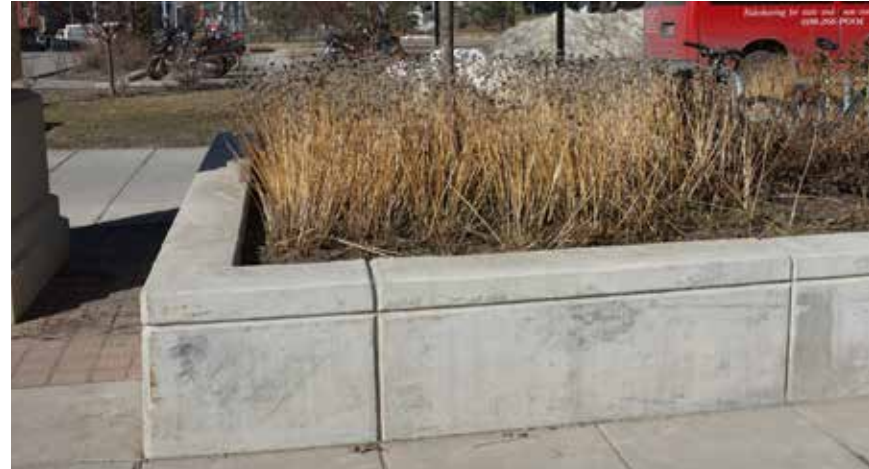
Figure 117 Architectural Concrete Wall Finish
