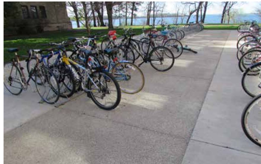
Figure 108 Pervious Concrete is Encouraged in Low Traffic Pedestrian Areas.
