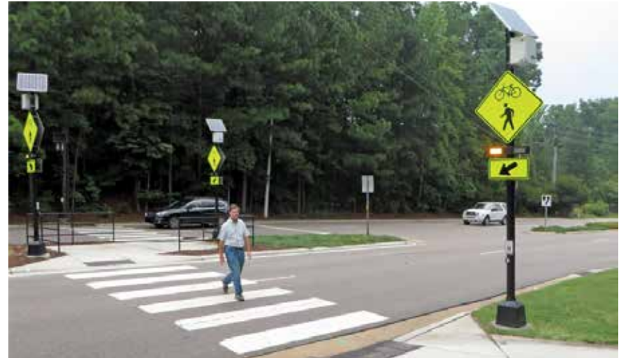
Figure 178 Rectangular Rapid Flash Beacon Assembly, Location Unknown
