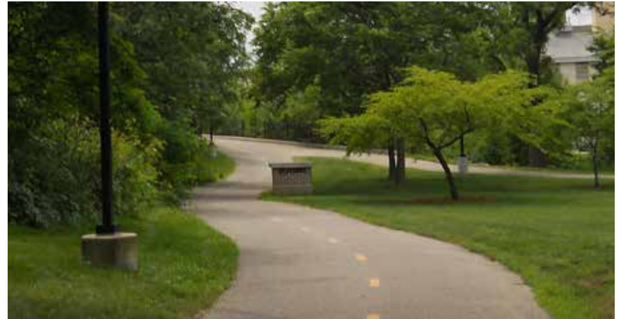
Figure 109 Multi-Use Pathway of Standard Asphalt Paving
