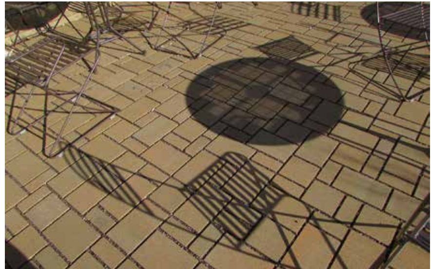
Figure 114 Pervious Pavers are Encouraged in Low Pedestrian Traffic Areas
