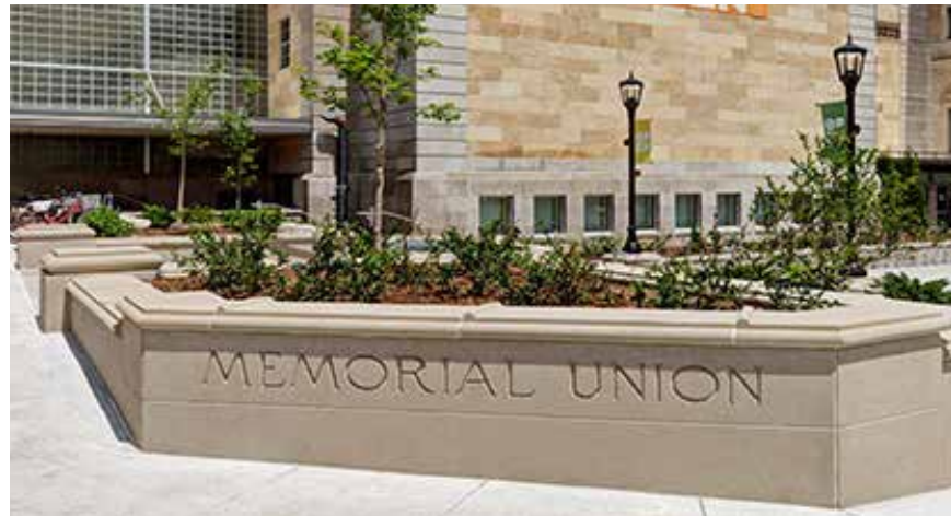
Figure 118 Precast Concrete Wall Finish
