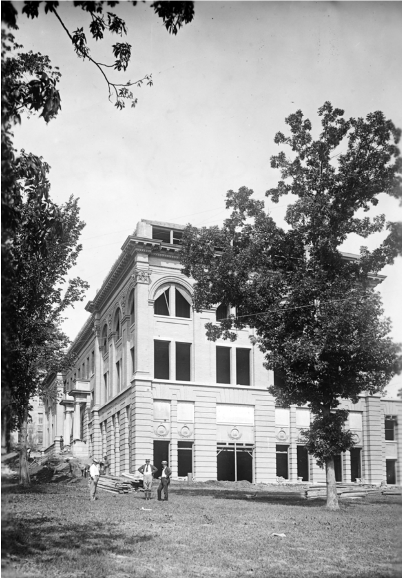
Figure 16: Engineering (later Education) building, looking northwest, ca. 1900.
