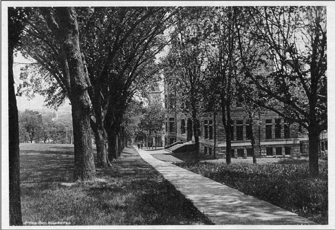
Figure 15: Law building, looking southeast, ca. 1898; razed 1963.
