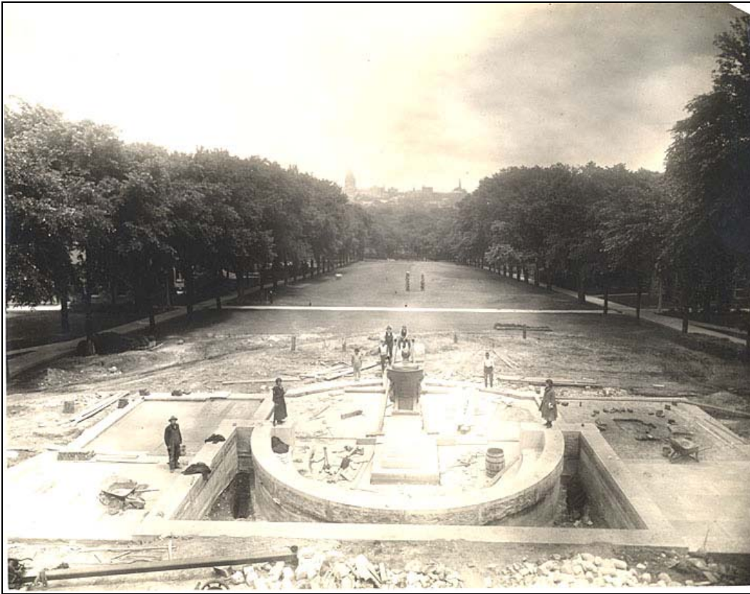
Figure 27: Lincoln terrace and exedra under construction, ca. 1918-19.
