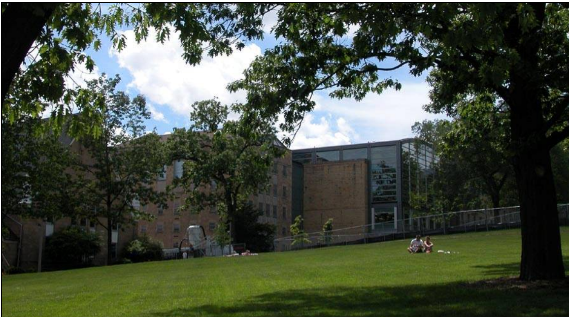
Figure 44: The most recent addition to the Law building juts out into the mall at an odd angle, 2004.
